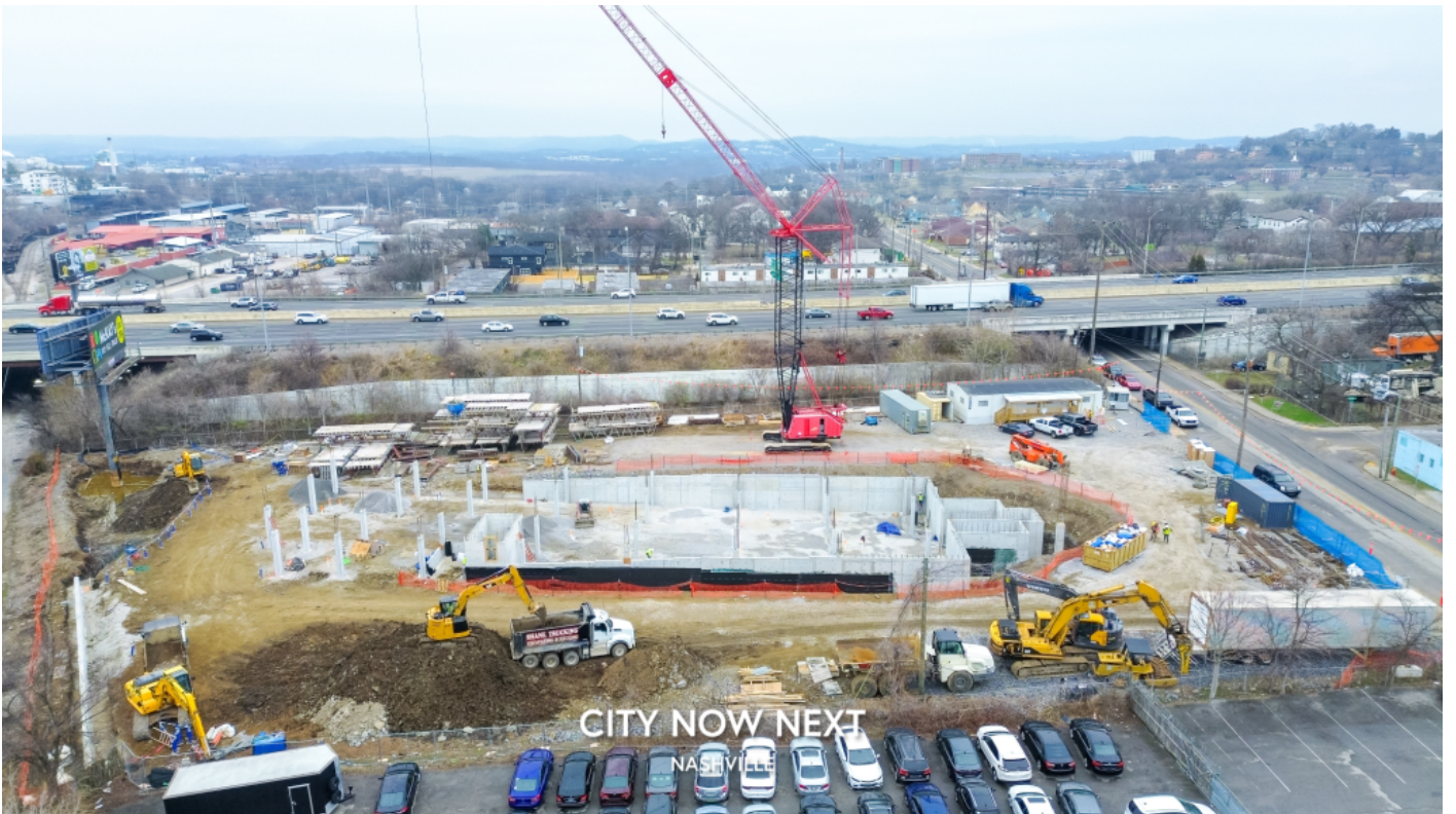
View facing Interstate 40.
