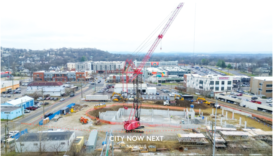
View facing Charlotte Avenue.
