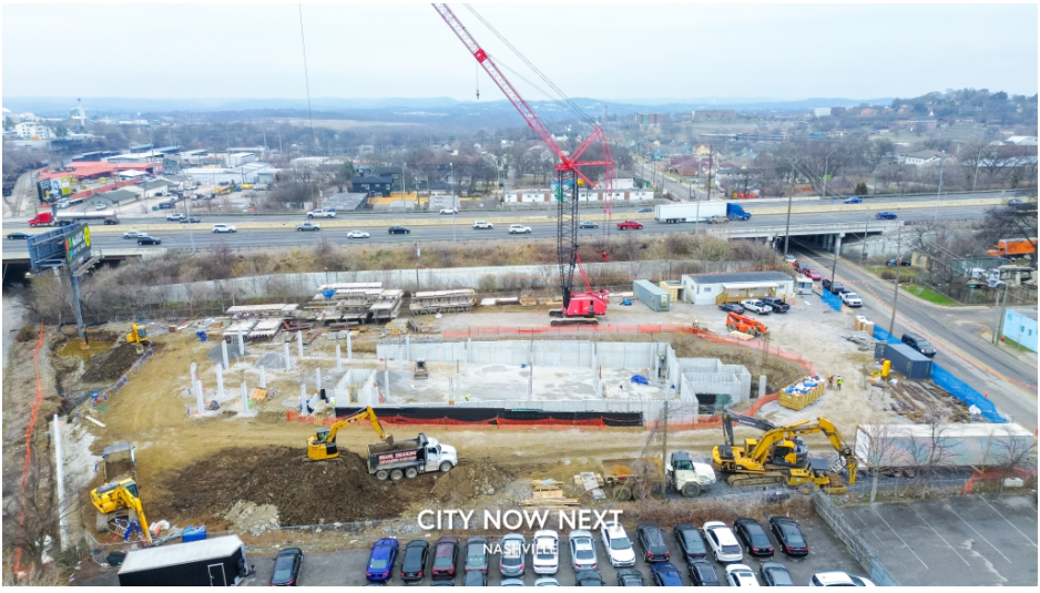
View facing Interstate 40.
